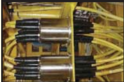
Example of Electrical Distribution Unit (EDU)
