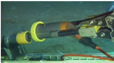
Figure 1: ROV Installation of Wet-Mateable Connector
