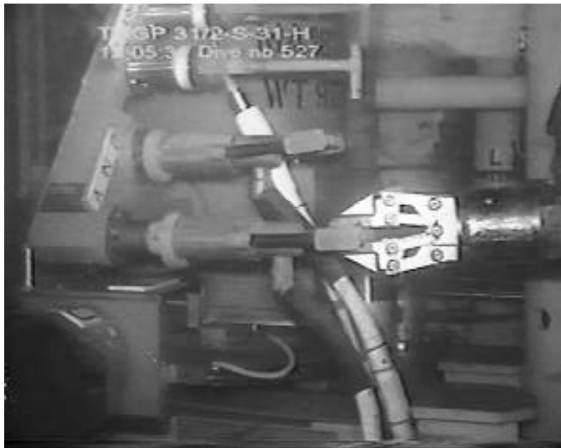
Photo 1: ROV Installation of Wet-mate Fiber-optic Connector
